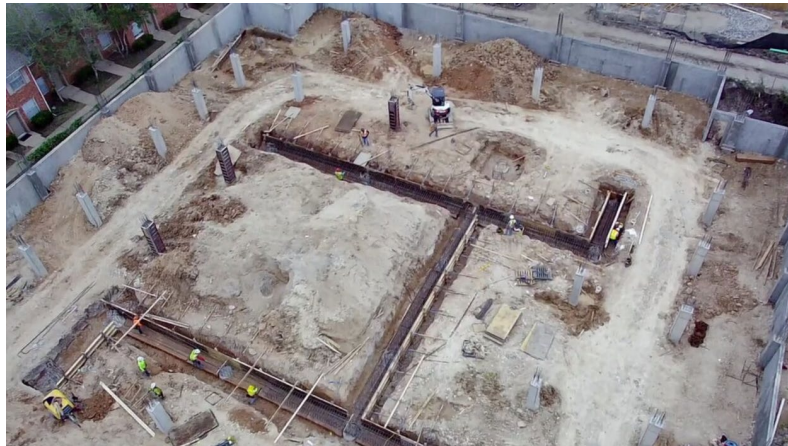
Construction as of October 12, 2023
