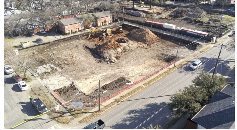
Construction as of January 5, 2023
