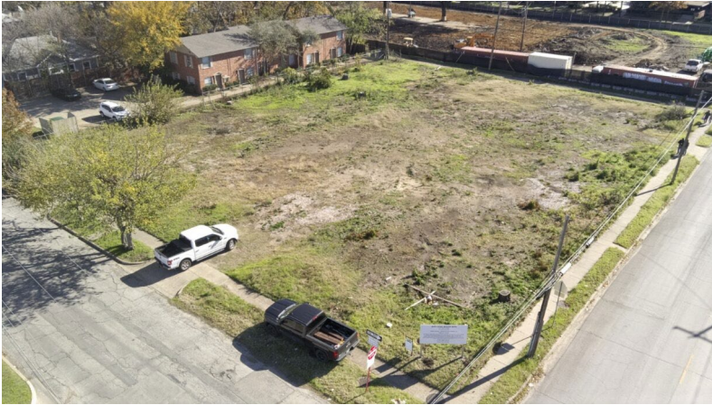
Construction as of November 30, 2022
