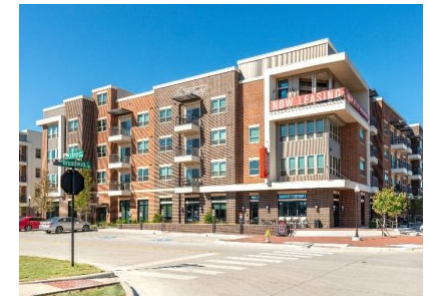
Switchyard | Carrollton, TX | 234 units 3
